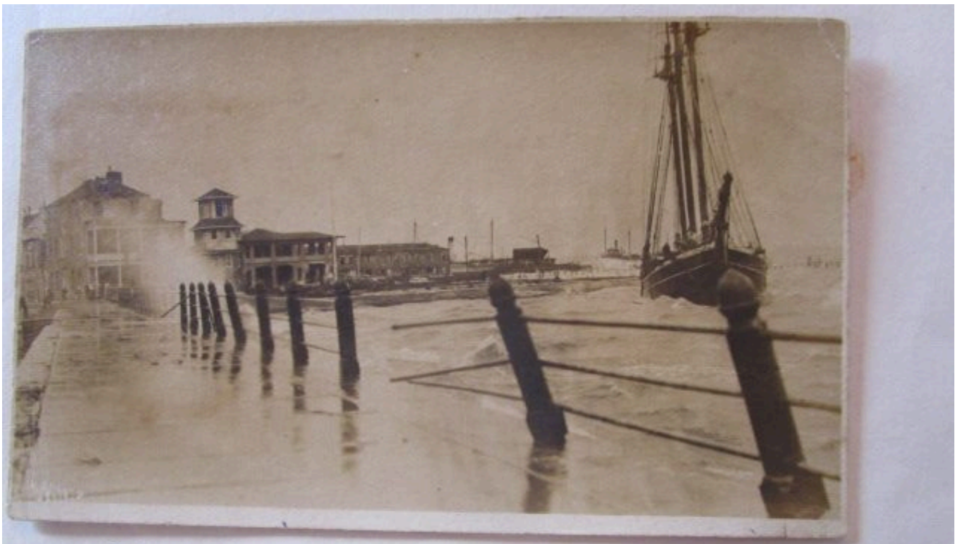
Storm of 1911 East Battery, Charleston, S. C.
